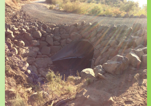
Left: Granite Creek tributary road crossing before culvert replacement, and Right: after culvert replacement.
