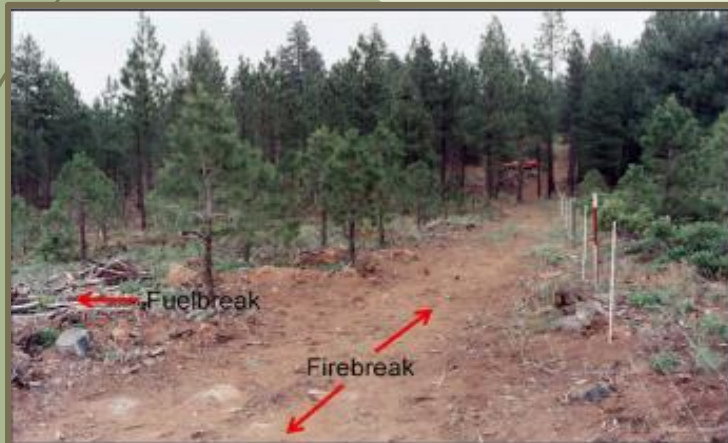
Figure 13a. A perimeter dirt road serves as a fire-break. The area immediately to the left is a fuelbreak where young pine have been thinned and flammable shrubs have been mowed.
